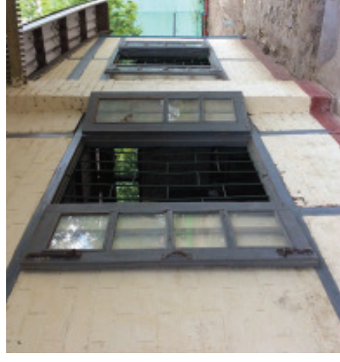
Building construction status: interior | Facade
