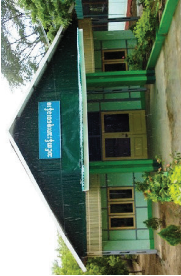
Typical workshop building Roof ridge / gable: Opportunities for ventilation: raise ridge cover / grill cover for gable
