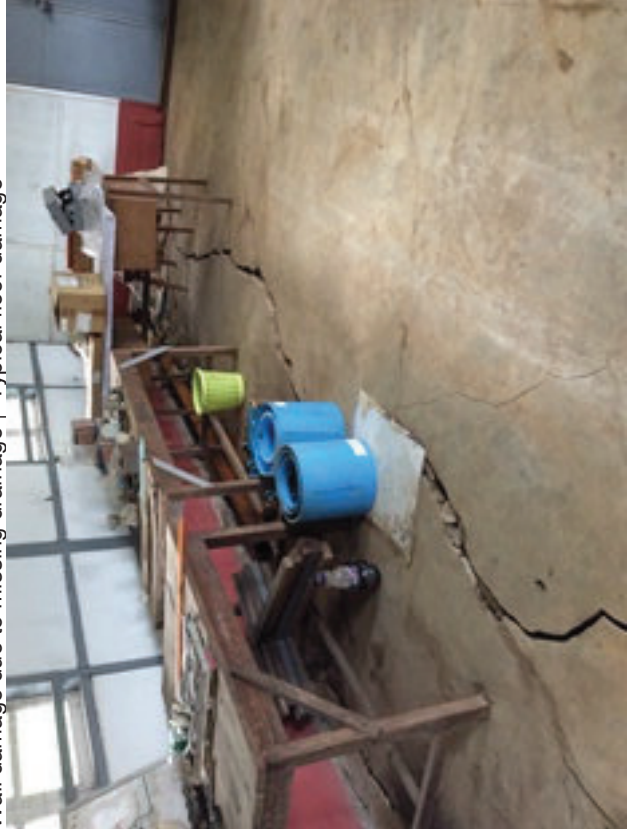
Wall damage due to missing drainage | Typical floor damage
