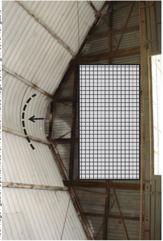
Typical workshop building Roof ridge / gable: Opportunities for ventilation: raise ridge cover / grill cover for gable
