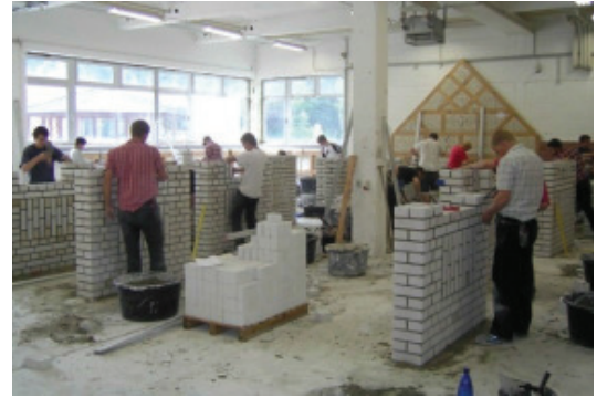
Trade testing for brick layers, work places separated by walls *7
