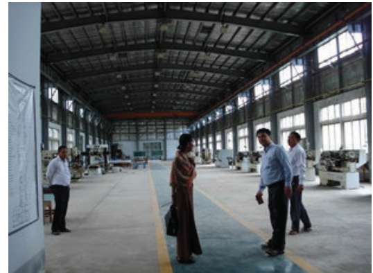
Existing workshop interior condition
